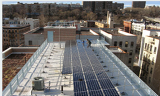
INSTALLING SOLAR IN NEWYORK CITY
