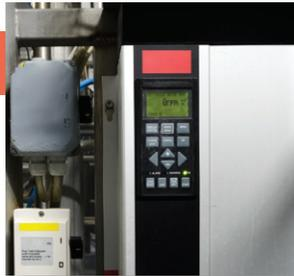
These systems are often designed in such a way that fans run at a constant speed, with their output controlled downstream by a mechanical valve. It's much more efficient to control the speed of the fan itself using a VFD.
