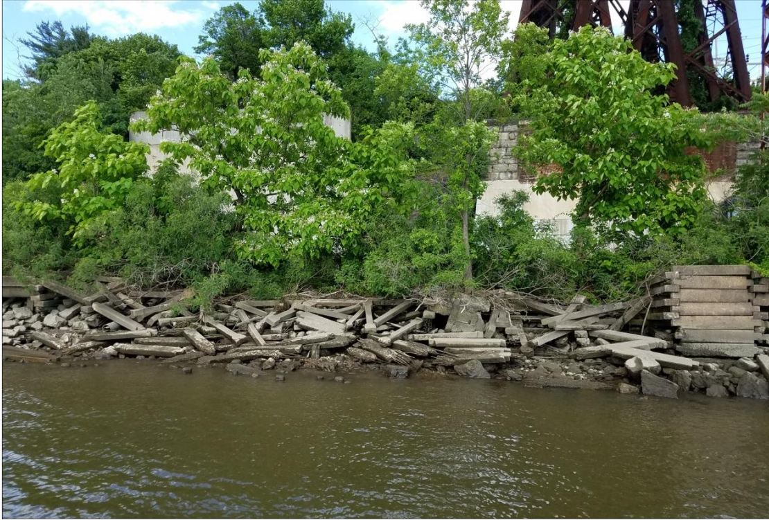
Photo 7 – Typical shoreline view of project area showing intact and deteriorated bulkhead; sideslope grading and capping will occur across this area
