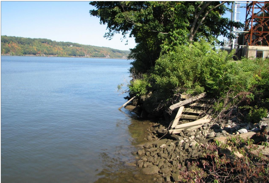
Photo 8 – Looking north along former MGP site shoreline; sideslope grading and capping will occur immediately along the shoreline and dredging and backfill work will occur approximately 100 feet offshore in the midground
