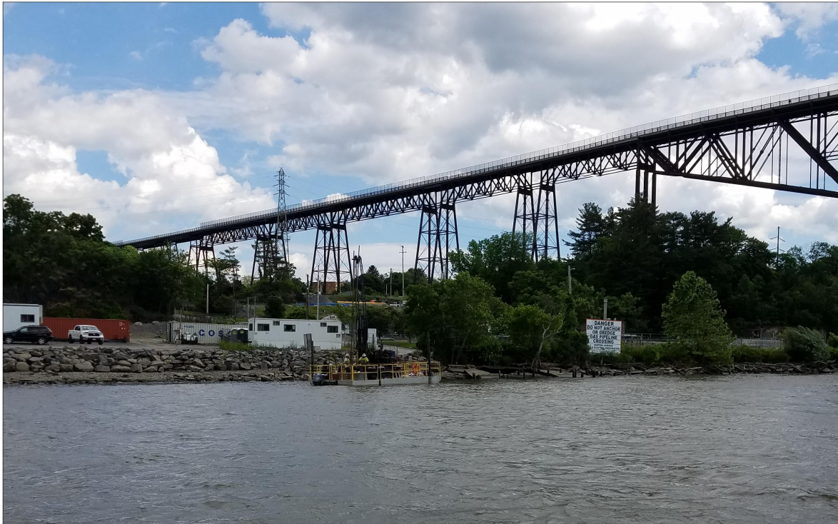
Photo 1 – Looking east across dredging area from river at northwest corner of former MGP and gas pipeline crossing warning sign. Note Walkway Over the Hudson Bridge crossing above
