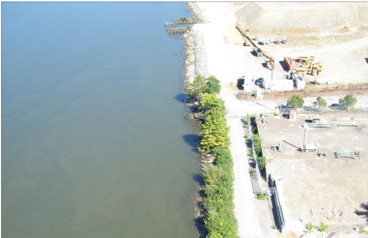
Photo 6 – Looking north from Walkway Over the Hudson showing where sideslope grading and capping will occur along shoreline
