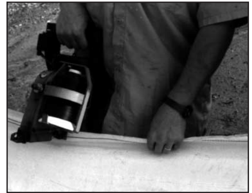
Figure 39 - Sewing Fabric Panels
