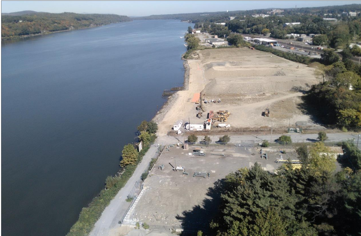
Photo 5 – Looking north from Walkway Over the Hudson; sideslope grading and capping will occur in foreground along shoreline from Dutchess Avenue (midground) southward and dredging will occur approximately 100 feet off shoreline to a distance of 500 feet north of Dutchess Avenue
