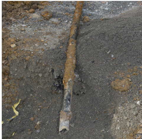
Central Hudson is replacing steel and cast iron gas main (left) with high density polyethylene plastic (right). The majority of these lines are located in the region's cities and villages, where gas service was first introduced in the early 1900s.
